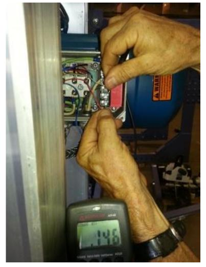
Using your multimeter, hold one contactor on the small red wire and the other contactor on the small white wire.
