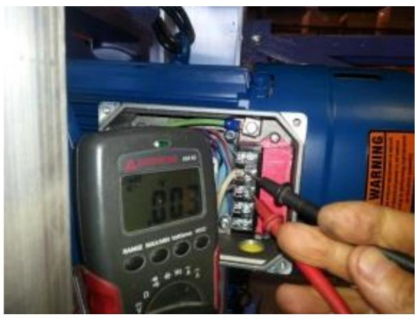
First, check main incoming power. The black and white wires, position 2 and 3. This should read 460v +/- a few volts. You do not need to loosen the wires, simply hold multimeter on the appropriate posts.
